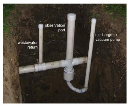
Figure 2-2. Photograph of Collection Vessel with Access Ports.
