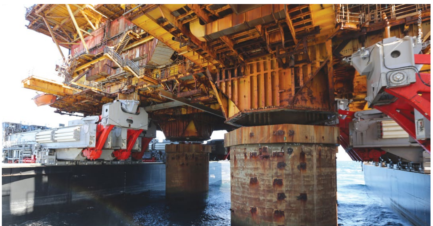
Fast lift of the Brent Delta topsides from their concrete legs
