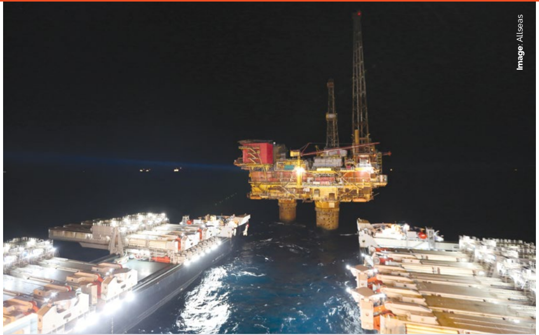
Pioneering Spirit moving in around the Brent Delta topsides
