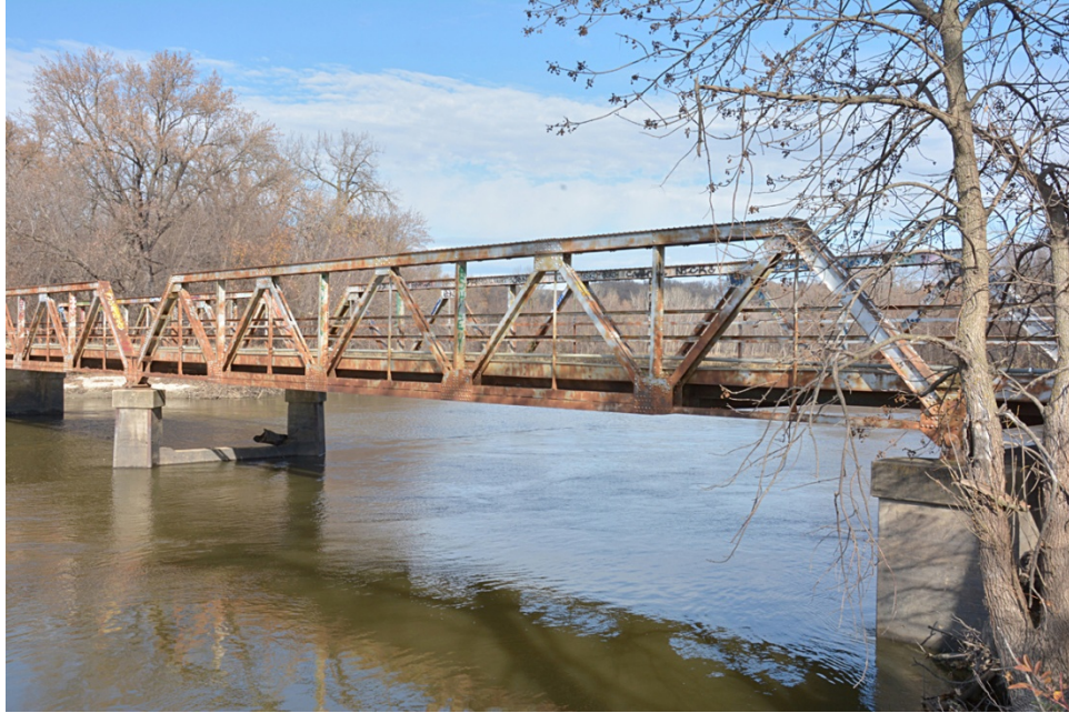
West side of south truss span (facing NE)
