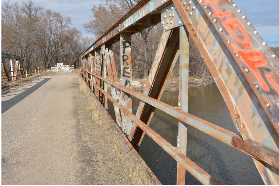
East truss with steel angle railing (facing N)
