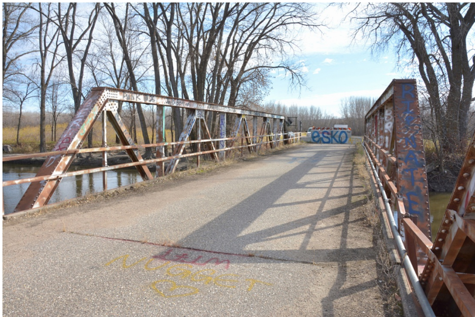
North end of south truss span (facing S)
