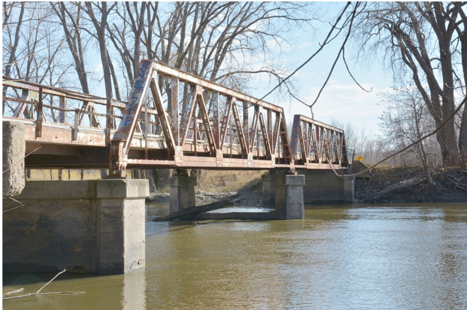
West side of the bridge (facing SE)
