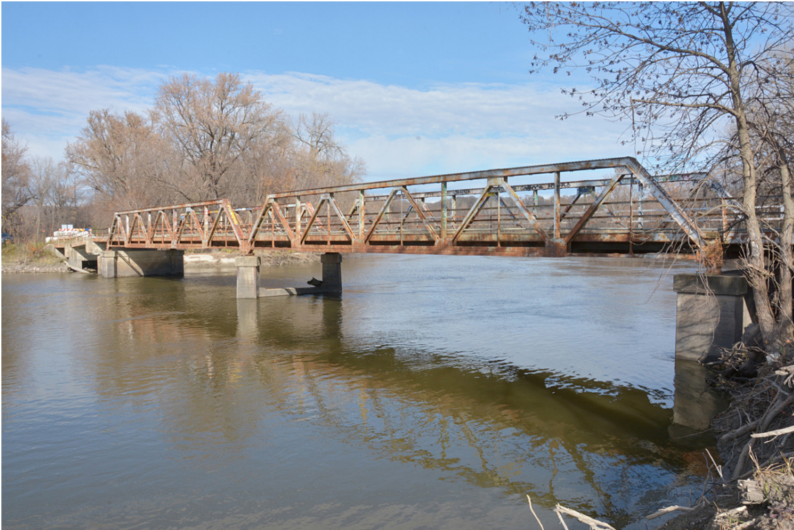
West side of the bridge (facing NE)
