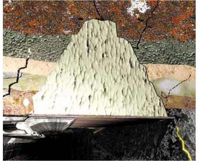
Cavity filling with MasterRoc MP 367 Foam
