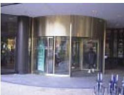
Figure 10 - Revolving door in the Mercy Hospital, Baltimore (USA)
