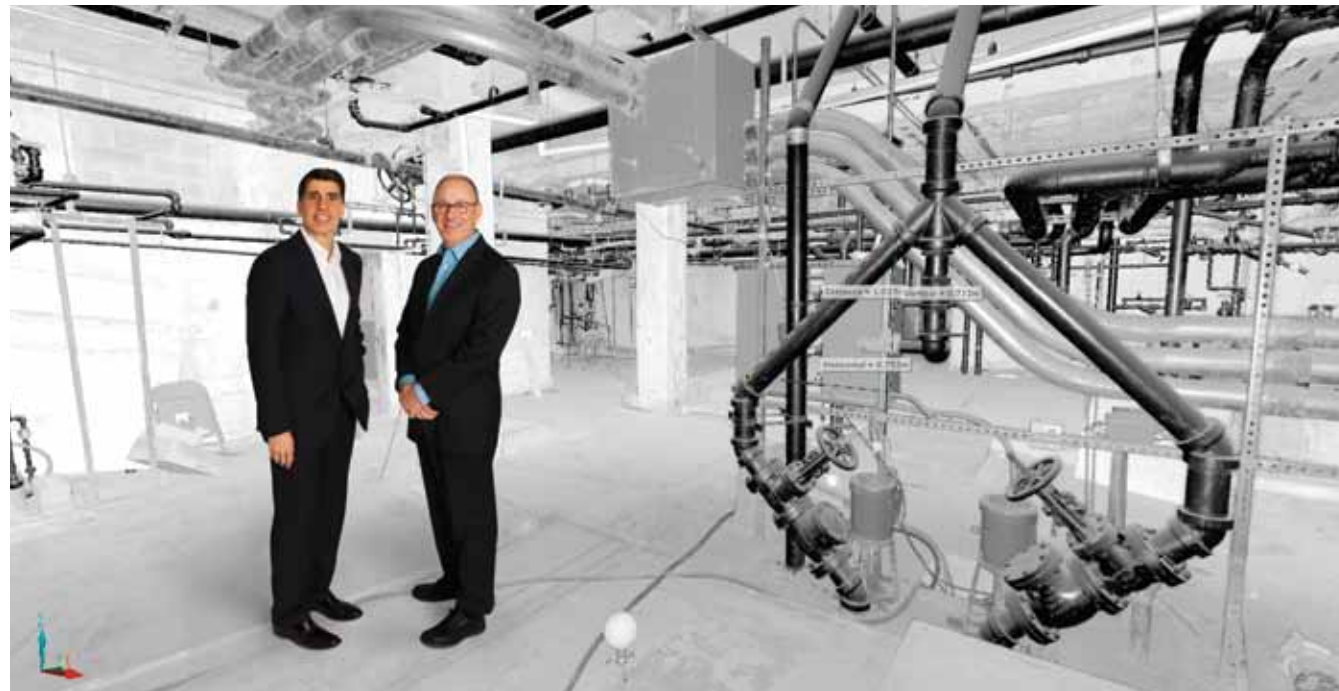
Tom Scarangelo and Bob DeScenza stand “in” a 3D laser scan of a New York hospital basement. We conducted the scan to establish baseline MEP data following CAT-90 Sandy. For more about our laser scanning capabilities, see pp. 10–11.
