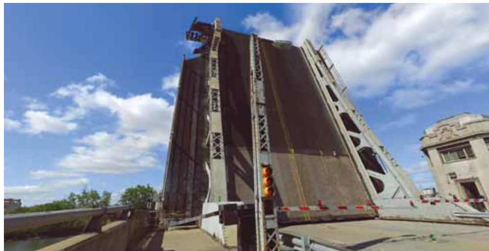
A photo (top) and point cloud rendering of a bridge damaged by a ship. The 3D model generated by the laser scanner can be used as the basis of a FIM that stores documents, photos and other information related to the investigation.
