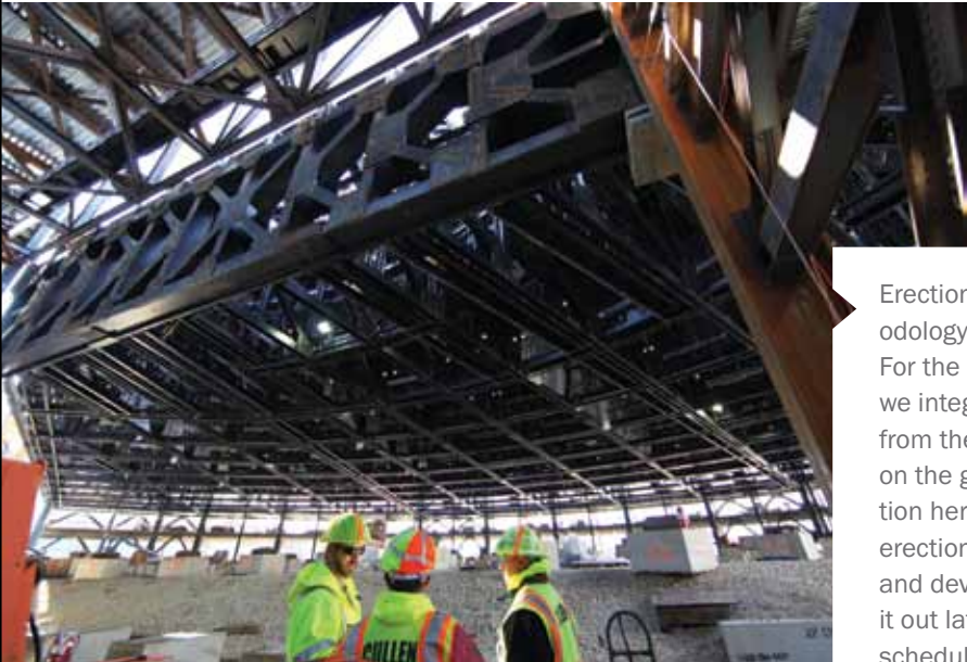
The 275-foot truss that supports the roof.
