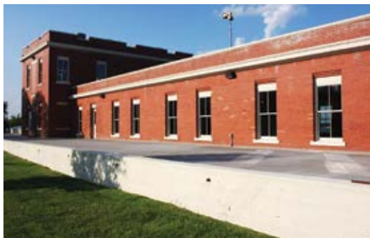
Filter Building exterior, after rehabilitation
