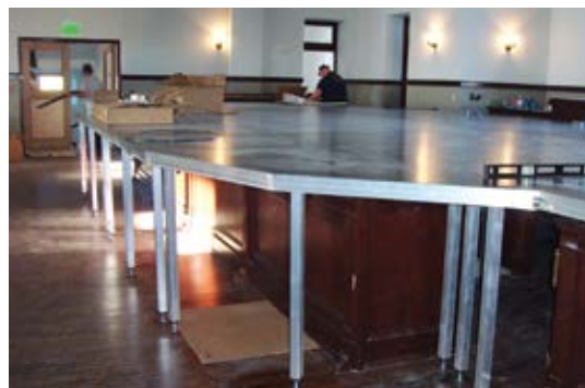
Aluminum-framed stage platform designed to fit over restored judge's bench and platform at the McKinney Performing Arts Center
