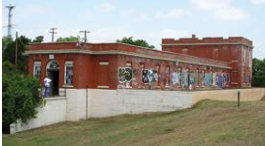
White Rock Lake Filter Building exterior, before reclamation
