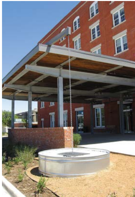
Rainwater harvesting at Nylo Hotel entry canopy
