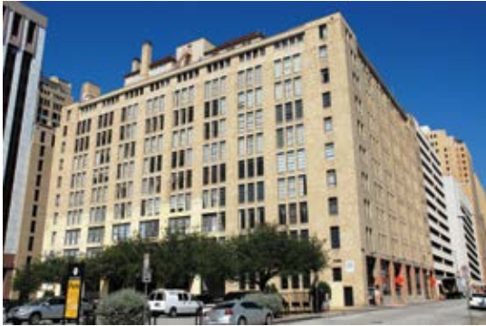
Exterior, former Santa Fe Warehouse Building No. 2
