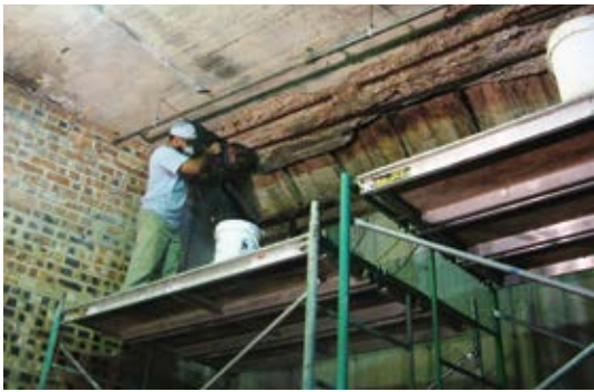
Extensive repairs in underground parking garage
