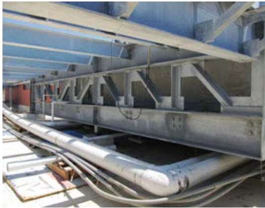
Galvanized steel truss supporting rooftop infinity pool and patio deck
