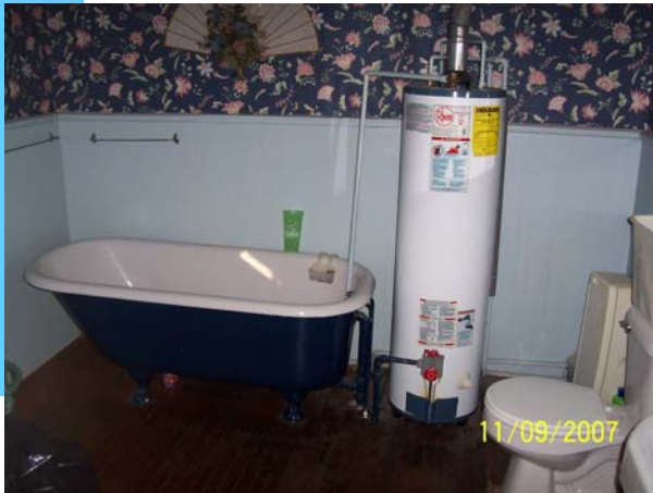
Good use of space. The release valve drains directly into the bath tub.
