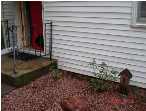
The little house looks leaky enough to be considered outside and not a separate Zone.
