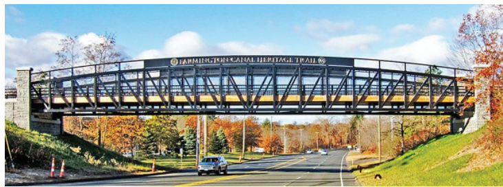
A bridge over Rt. 6 on the Farmington Canal Heritage Trail.
