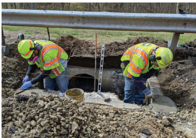
Joe Lynch and Julio Alicia rebuilding a catch basin for a VIP.
