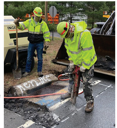
Masked crew works on a catch basin replacement in Avon.
