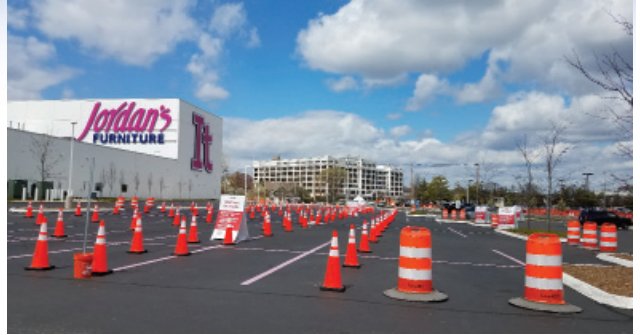
Quickly completed CVS Testing facility in New Haven. See details.
