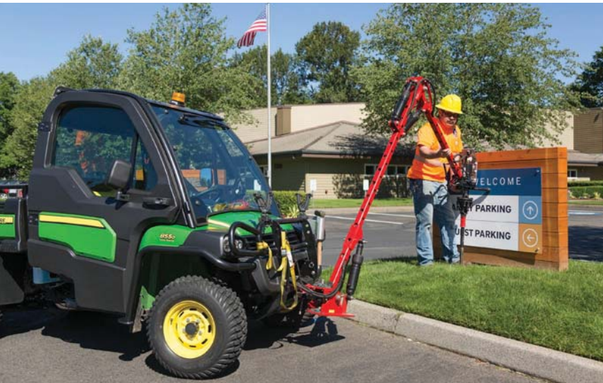
In this picture we have a common situation where a business puts up a new sign right next to our valve but does not understand the room needed to access it. A standard valve wrench would not clear the sign but can easily be exercised with our automated valve turner.
