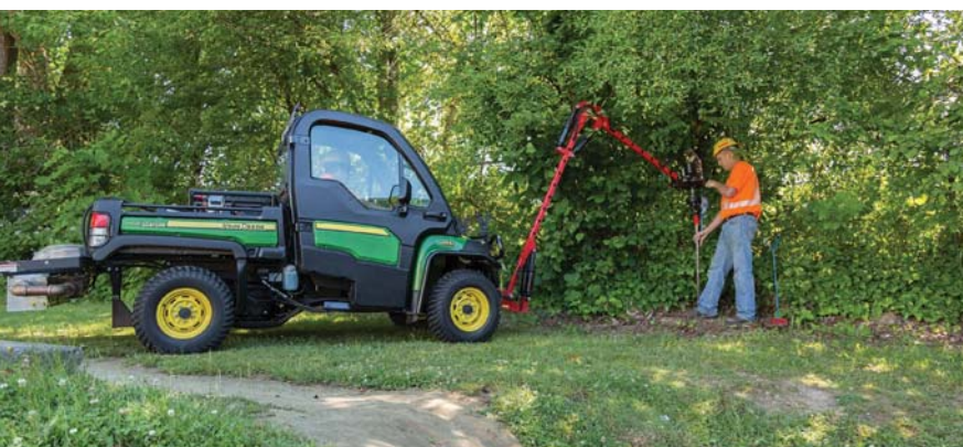
Another example of a valve that's too close to a fence. A truck mounted turner would not be able to access the cross country main either.
