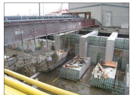
Rebuilding electrical vault lids.
