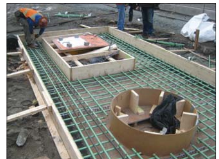
Rebuilding electrical vault lids.
