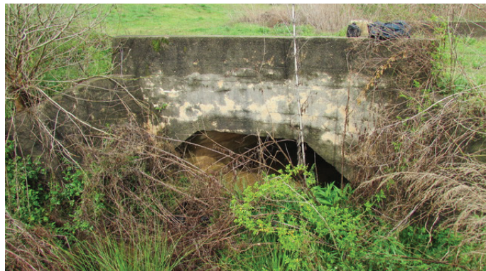
Figure 3: Detail of the old bridge. (Photo by Lamar Nelson)
