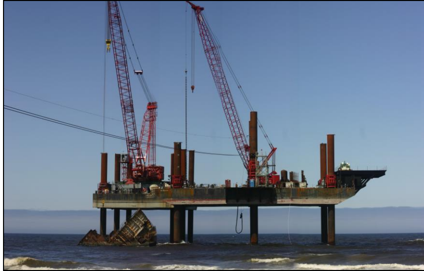
Barge with cranes held aloft on jacks.
