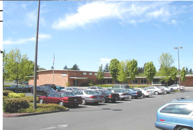
Figure 7-5.2.2 Inspection and Testing For
