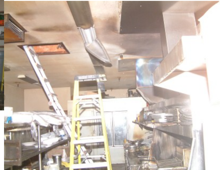
Sprinkler contained fire that escaped kitchen hood
