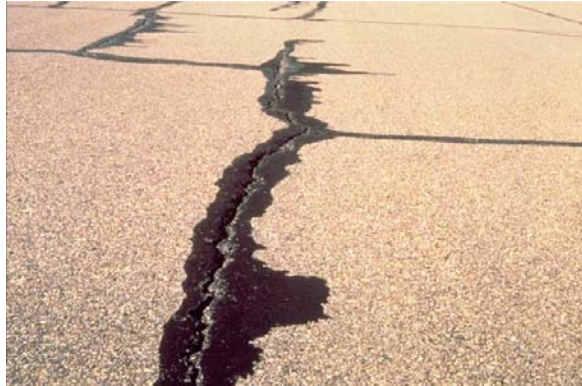
Photo 13. Excess sealant.
