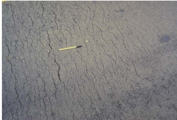
Photo 31. Checking under steel wheel rollers.
