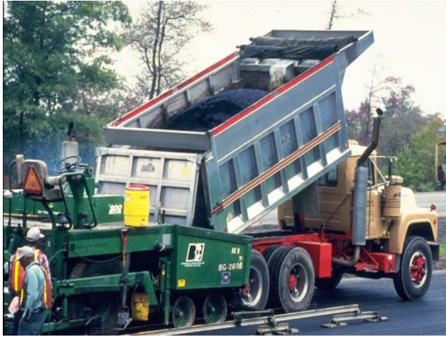
Photo 16. Dumping directly into paver.
