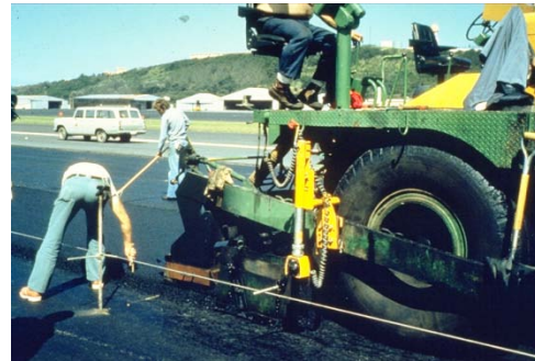
Photo 24. Use of stringline to control grade.
