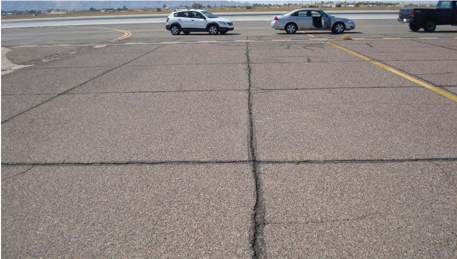
Photo 28. Reflective cracking.
