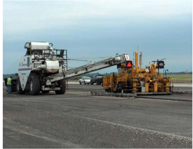
Photo 17. Use of material transfer vehicle.
