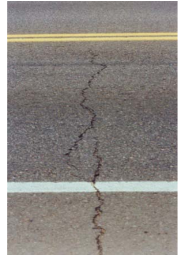
Photo 29. Reflective cracking.
