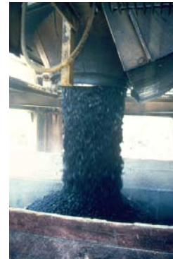
Photo 9. Dropping asphalt in small batches.
