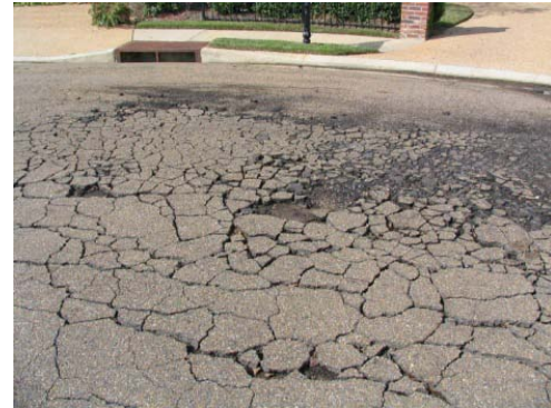
Photo 34. Alligator cracking.
