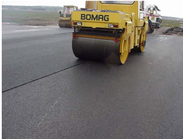
Photo 22. Rolling longitudinal joint.
