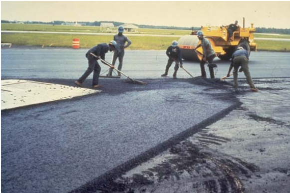
Photo 20. Excessive handwork.
