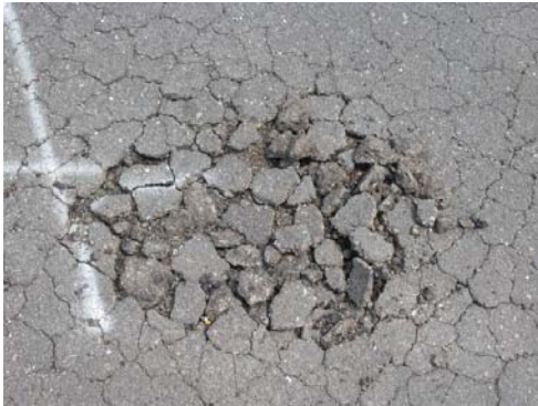
Photo 33. Alligator cracking.
