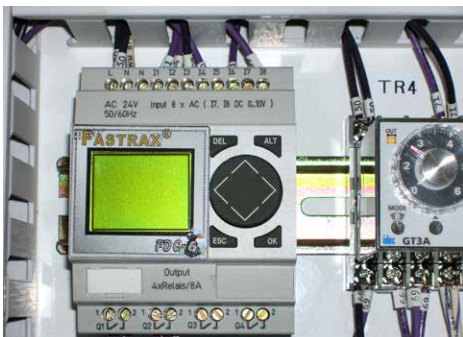
Figure I.1.1 - FDC-6/FDC-7 Integrated Control & Sensor System
