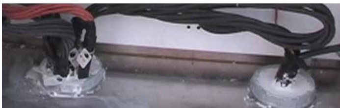
Figure G.6.2 - Sealed Conduits
