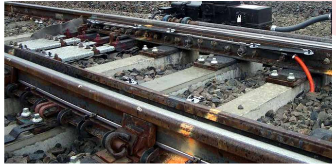
Figure E.4.3 - Track Switch Construction
