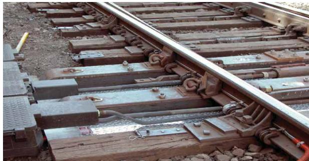
Install clamps on rear heater every 2".
