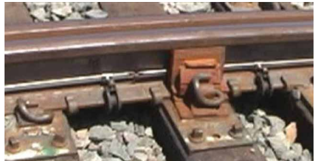
Install the second heater from the rear of the switch so that the point of the rear heater meets the point of the front heater.
