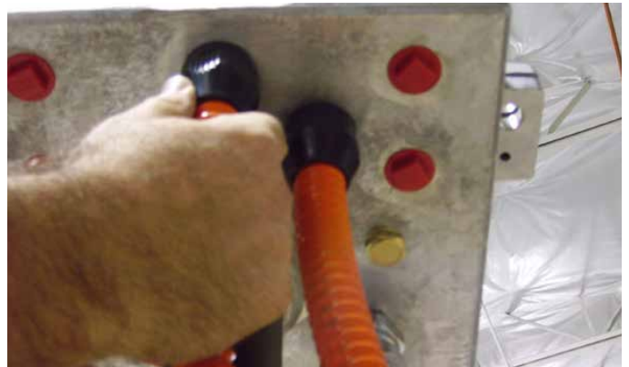
Figure E.3.4 - Install Orange Conduit to Junction Box
