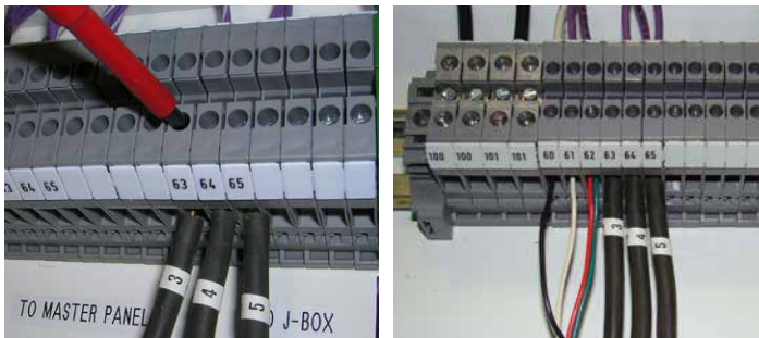
Figure G.6.1 - Snow Sensor Wiring
