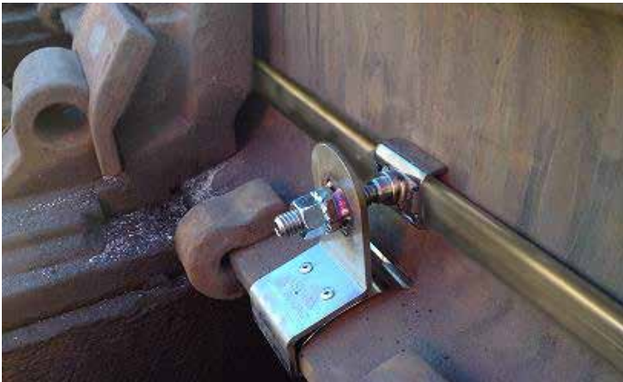
Figure E.1.1 - Heater Installed with FRB600 spring rail clamp
