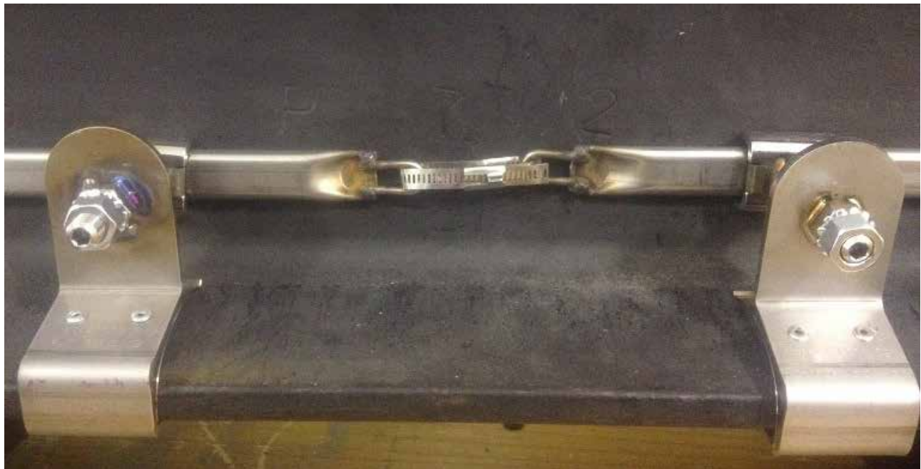
Tie the heater dead ends together with a stainless steel wire tie.
