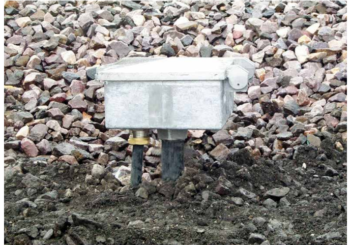
Figure D.1.8 - Junction Box Installed
