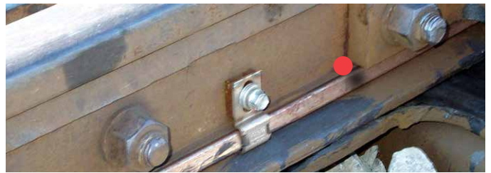
Figure E.6.3 - SwitchBlade® heater clamp installed *Look for proper clearance
