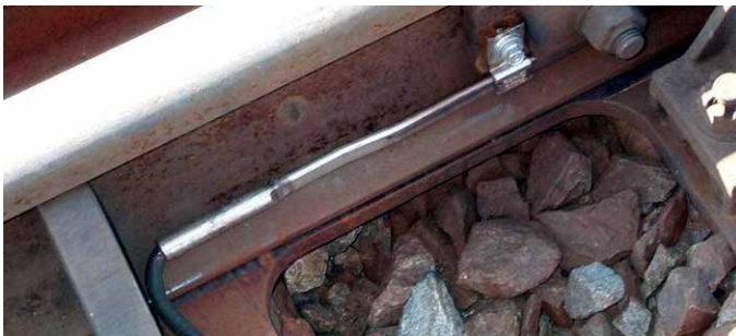
Figure E.6.2 - SwitchBlade® heater end clamp
