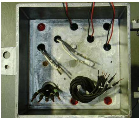
Typical Junction Box Cable Entries and Connections
