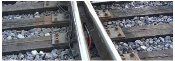
Figure E.5.1 - SwitchBlade® heater installation location
