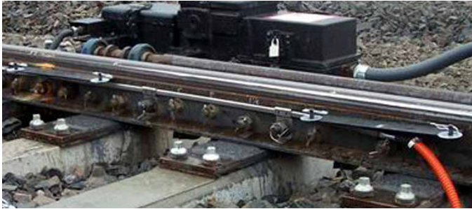
Figure E.4.1 - SwitchBlade® Heater and Spring Clamps
