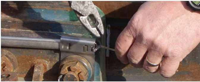
Figure E.4.5 - SwitchBlade® Heater End Tie-off
