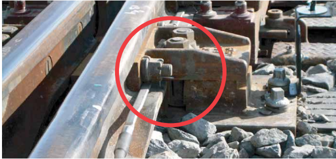
Figure E.7.1 - SwitchBlade® heater installed on frog wing rails
