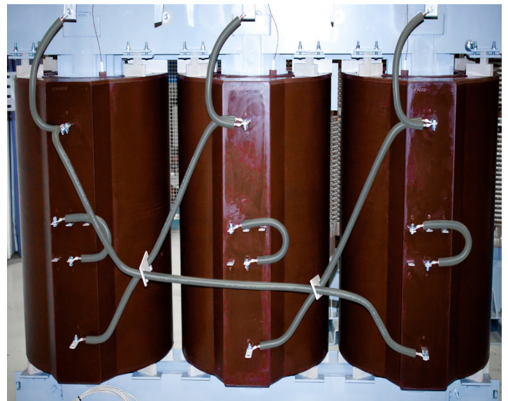
Cable connection - Delta primary
