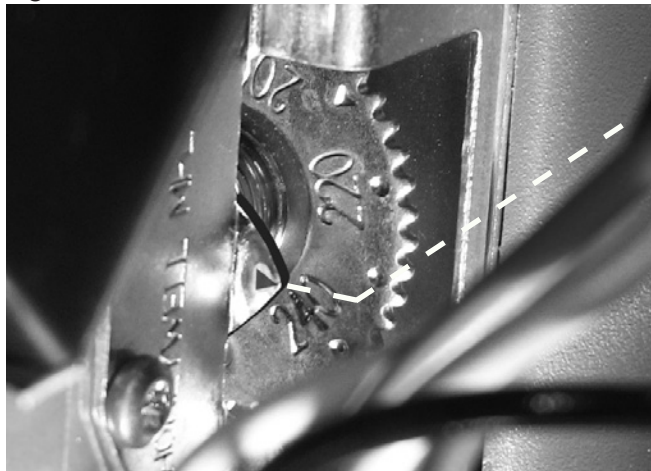
Figure 18B. Secondary, mechanical high-limit aquastat
