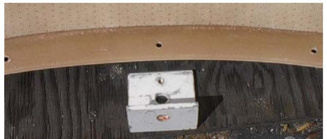
25. Attach three more brackets, in the same manner, so that the lifting brackets are in four equidistant points around the perimeter of the bottom flange of the lower panel assembly.
