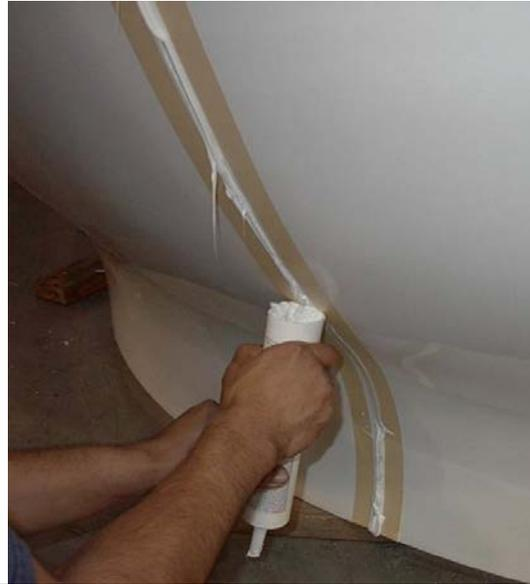
19. Repeat caulking, closing and cleaning the vertical flanges until all of the lower panel seams are closed.
