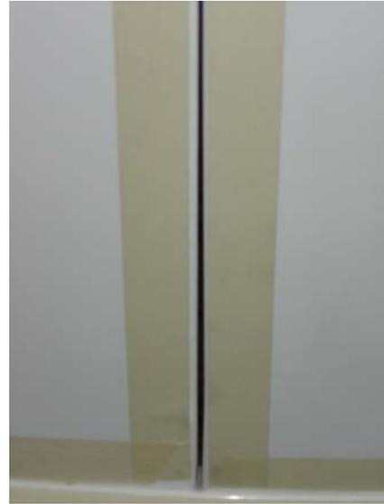
**NOTE:** It is extremely important to assure that the flanges are properly aligned before the bolts are tightened and kept in alignment as the hardware is aligned. This is necessary for the inside clearance and the outside aesthetic appearance of the radome. Please note this picture shown good alignment as observed from inside the radome and below a flange with bad alignment.
