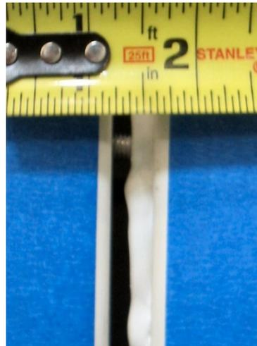
18. Clean excess caulking off of the flange area (inside and out). The empty caulking tubes can be used to clean off the excess caulk without scratching the radome finish.
