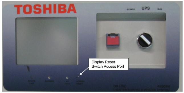
Figure 9-3 Display Reset Switch
