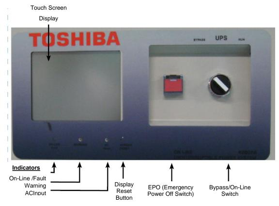
Figure 9-1 Panel Layout for Touchscreen Display
