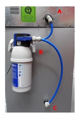
If your machine is **not** fitted with a base cabinet, the filter must be located in a suitable place such as below the counter or a nearby cupboard. It can be mounted in any orientation.
