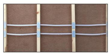
Allow 1/8-inch slack per foot of installed tubing.
