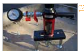
13 Conduct a pull test using the Hydrajaws testing kit to 6kN.
