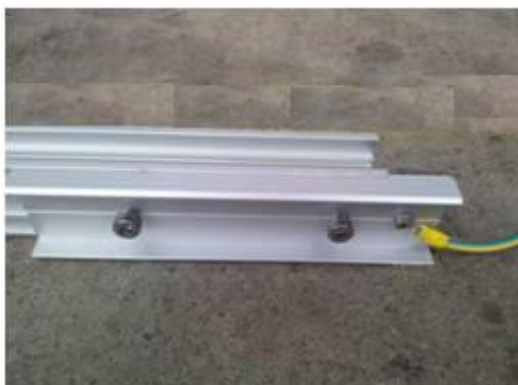
Rail splice attached to rail with both Allen head bolts
