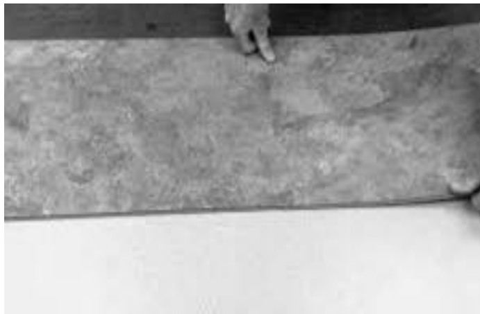
Square Cut Glue Down Installation
