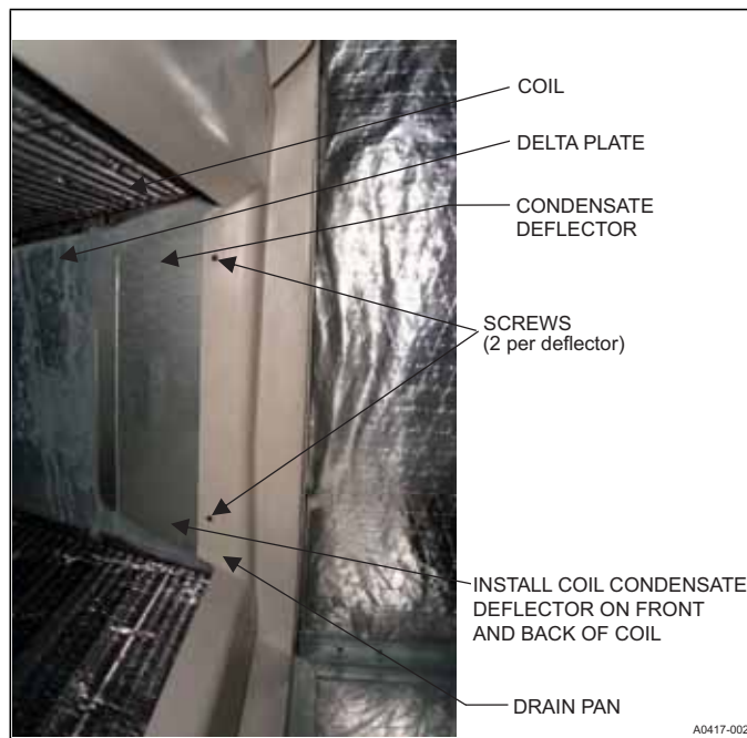
FIGURE 15: Coil Condensate Deflector Installation
