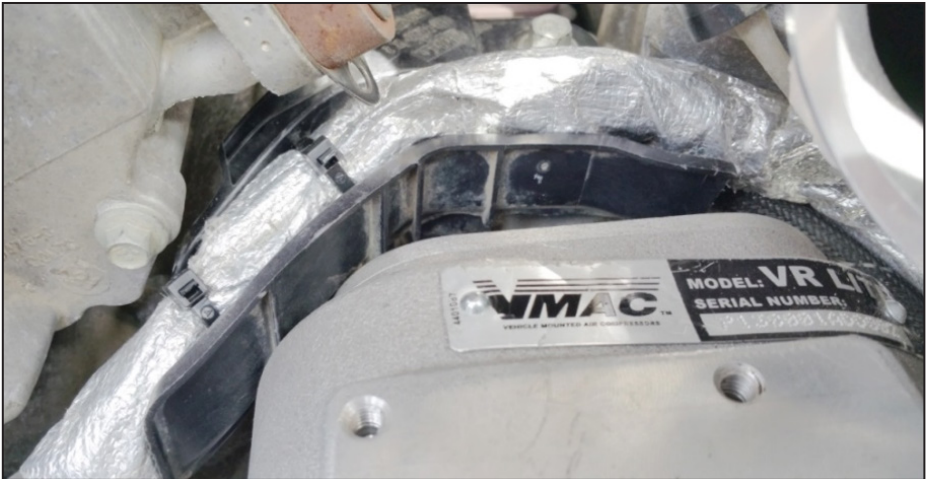
Figure 16 — Installing the cable tray (V300011 compressor shown)
