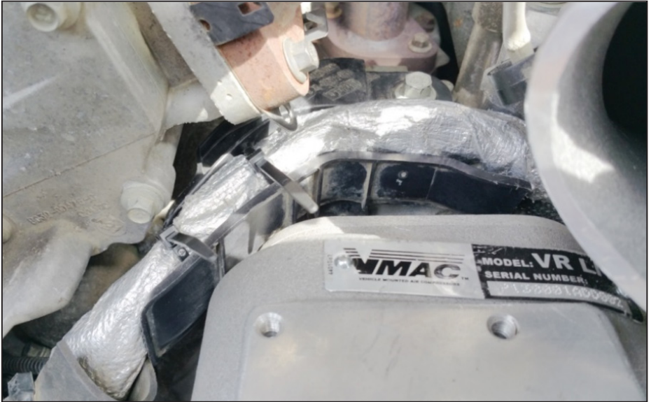
Figure 15 — Installing the cable tray (V300011 compressor shown)
