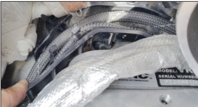
Figure 14 — Installing the cable tray (V300011 compressor shown)
