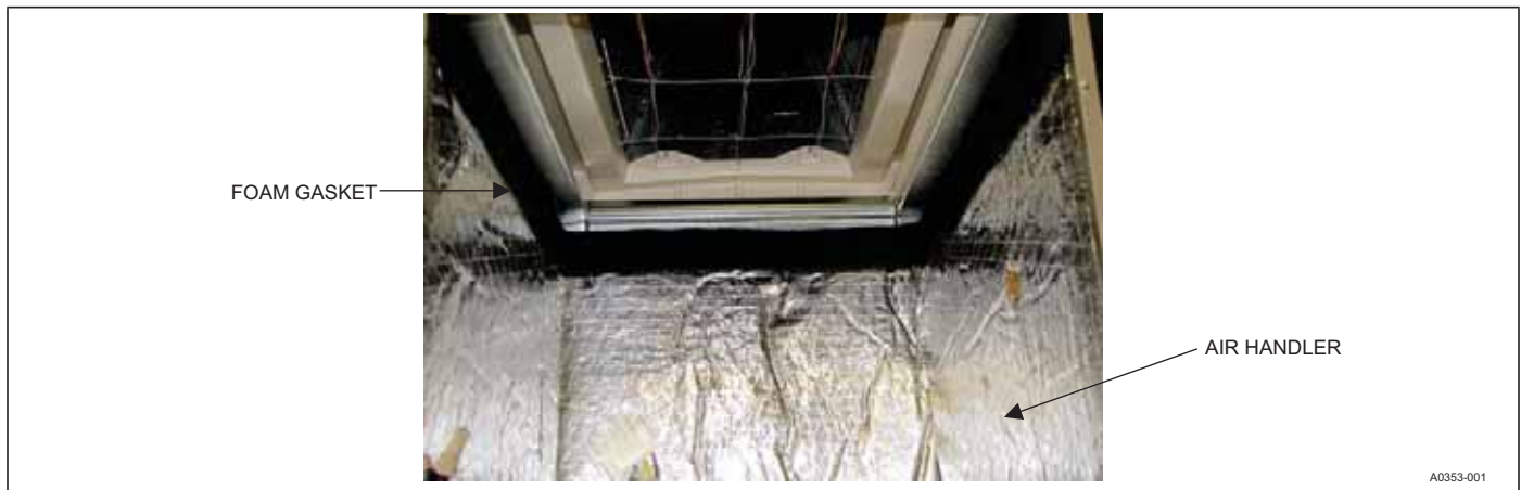
FIGURE 4: Gasket Location
