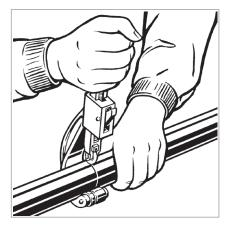
Cut the tube square using a displacement-type cutter or fine toothed saw.
