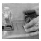
Remove faucet Spout first. Position both thumbs on the back edge of the lever and push forward.
