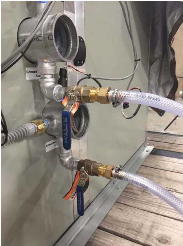
Figure 50. Typical setup for clean in place
