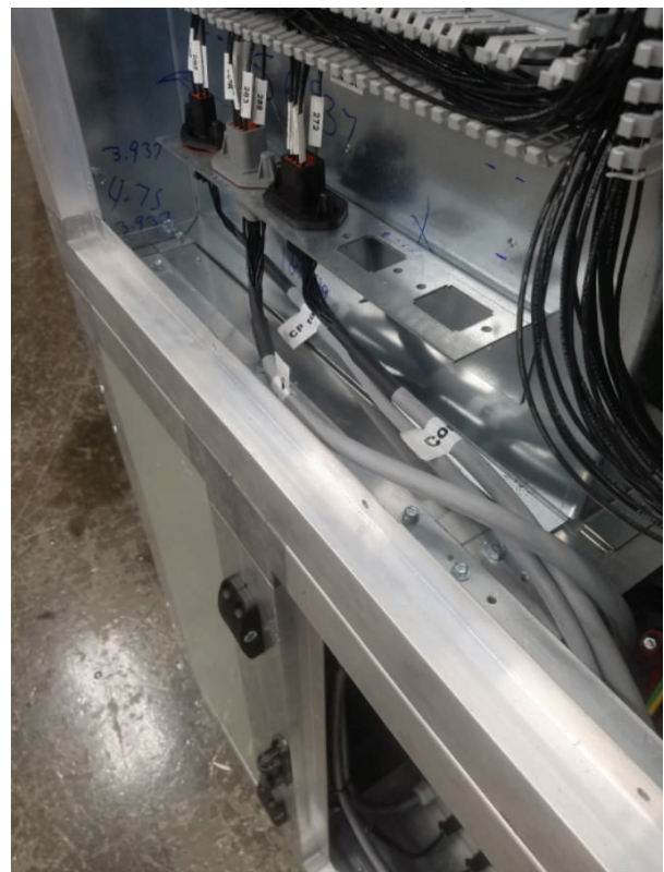
Figure 21. Compressor communication terminations
