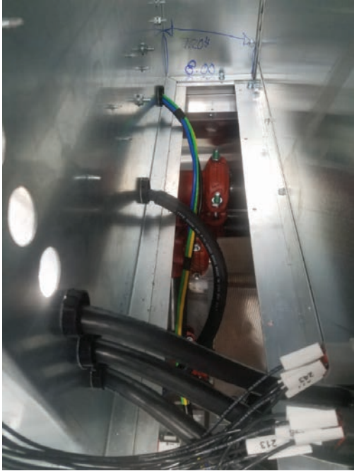
Figure 23. Compressor power terminations
