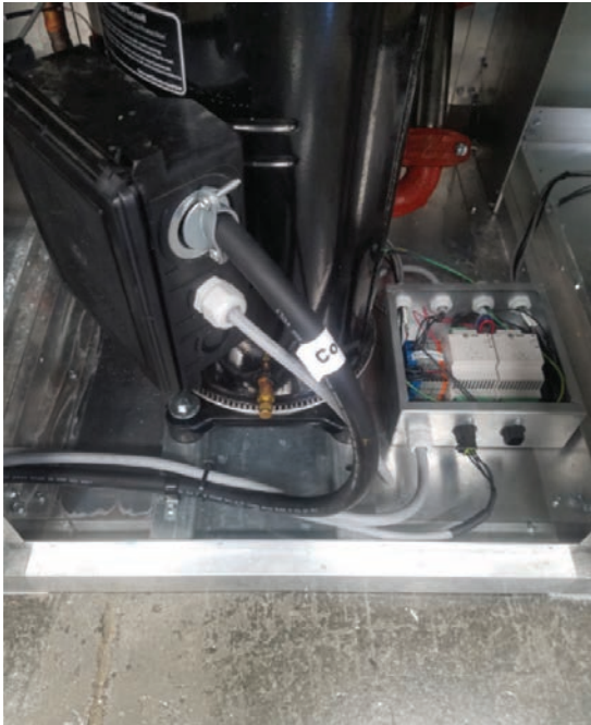
Figure 19. Variable speed power and communication wiring
