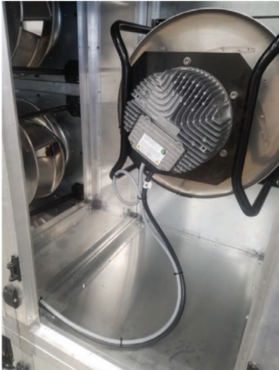
Figure 26. Fan power and communication wiring
