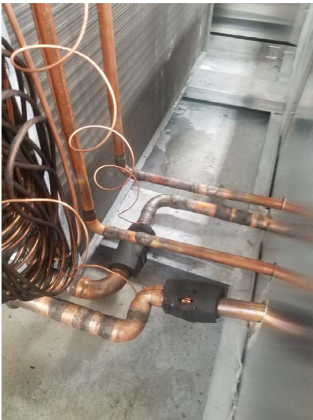
Figure 17. Braze suction and liquid lines
