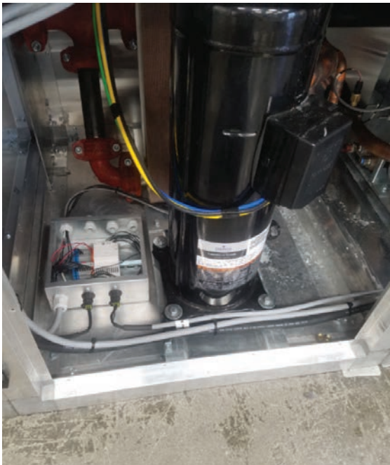
Figure 19. Variable speed power and communication wiring
