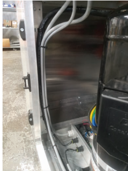
Figure 21. Compressor communication terminations
