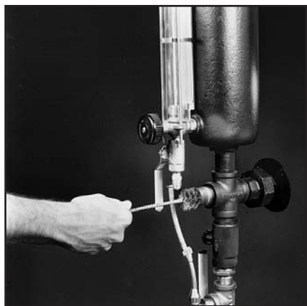
Remove cap at cross section; clean nipple to boiler
