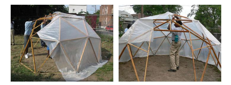
**step 28: Keep Adding Plastic Until Finished** Repeat the process until the dome is covered. You will need to put a ladder inside the dome to staple the plastic onto some of the top parts (see photo).
