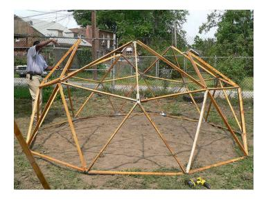
step 15: Connect The Top of the Pentagon At the top of the pentagons, attach a "B" piece to the 6-way connectors between each pentagon. Repeat until the five "B" pieces connected at the top of each pentagon form a pentagon.
