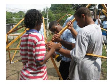
step 14: Connect The Bottom of the Pentagon Now attach "B" pieces between each pentagon at the bottom of the dome using the two 4-way connectors. Repeat until there are ten sides on the bottom of the dome.
