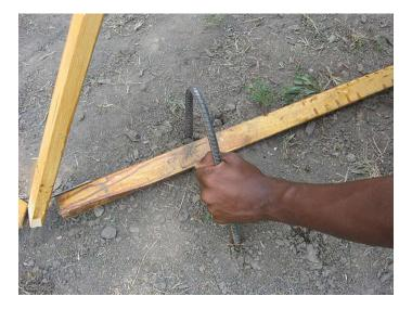
step 25: Anchor The Dome To The Ground With your drill hammer (small sledge hammer), hammer two pieces of rebar over each "B" piece into the ground. There are ten sides to the bottom of the dome, so you will use twenty pieces of rebar to hold it down.
