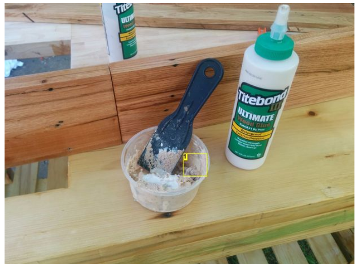
Image Notes 1. 50/50 mixture of sawdust and wood glue makes for a good filler.
