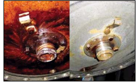
Vessel cover contaminated
