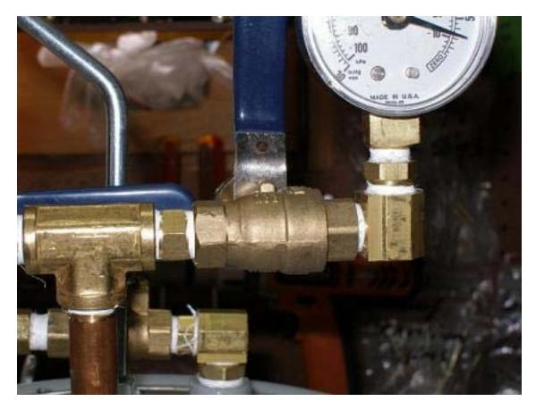
Now the right side, out of the ball valve, 1/4" elbow with female pointing up, 1/4" to 1/8" adapter, to vacuum gauge.
