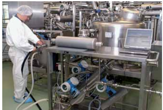
On-site calibration of flowmeters, pressure, temperature, analysis instruments, using mobile flow rig
