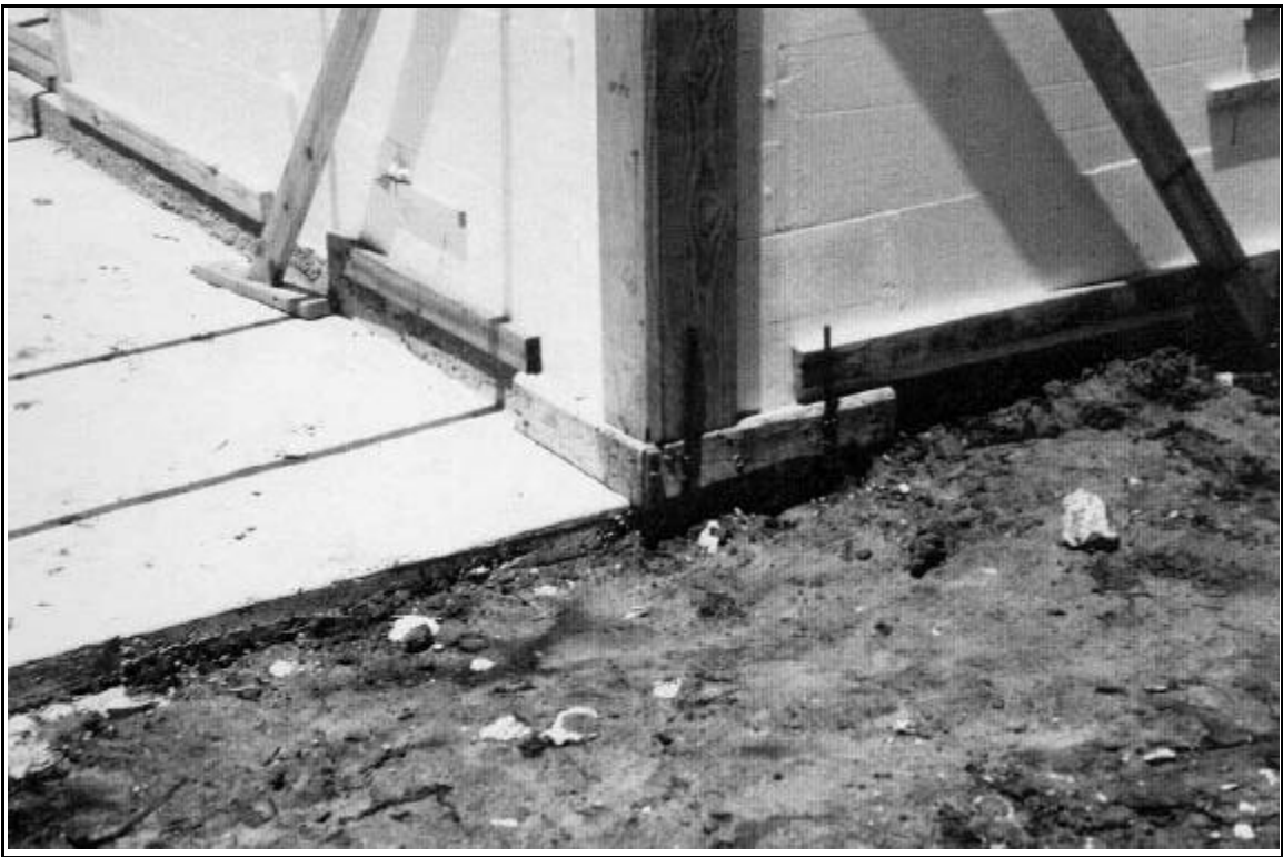
Photo 4: Site #1 - Corner Detail
