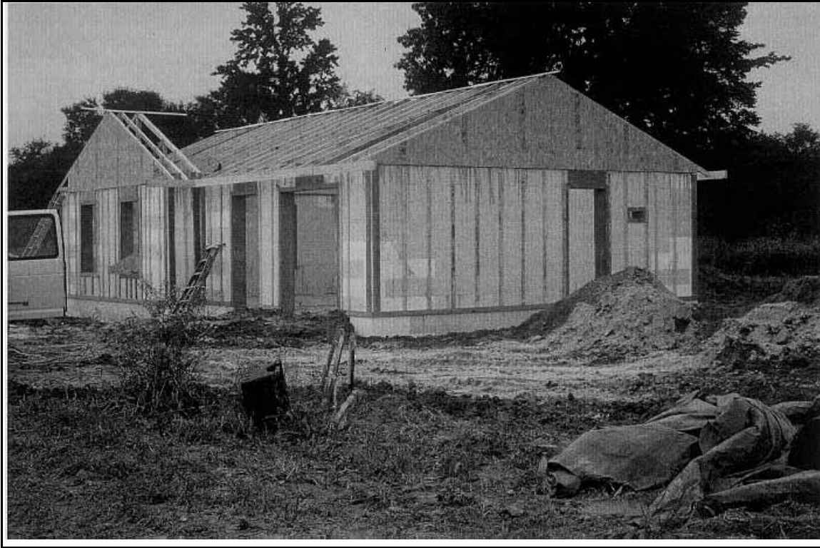
Photo 54: Site #4 - Unfinished Exterior and Roof Details
