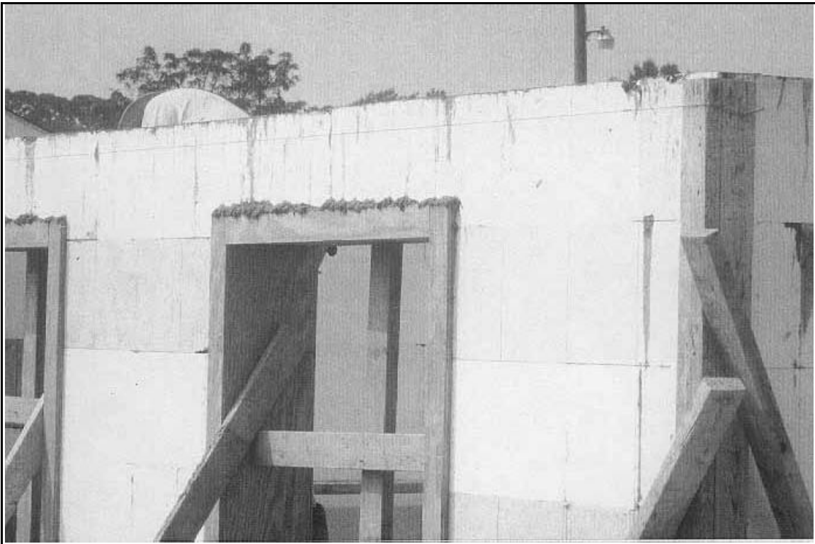
Photo 50: Site #4 - Window and Corner Detail
