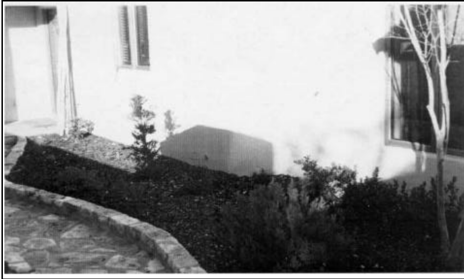
Photo 24: Slab Edge From Outside Under Natural Conditions
