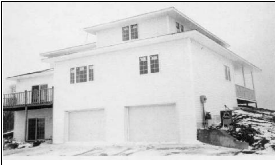
Photo 27: Site #3 - Rear Elevation
