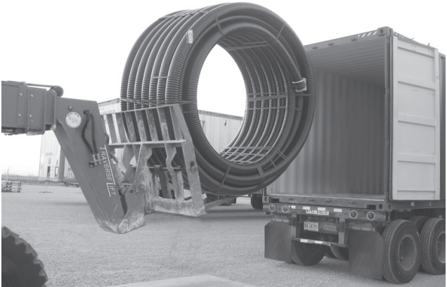
Fig. 4.1: Unloading INSULPEX with forklift
