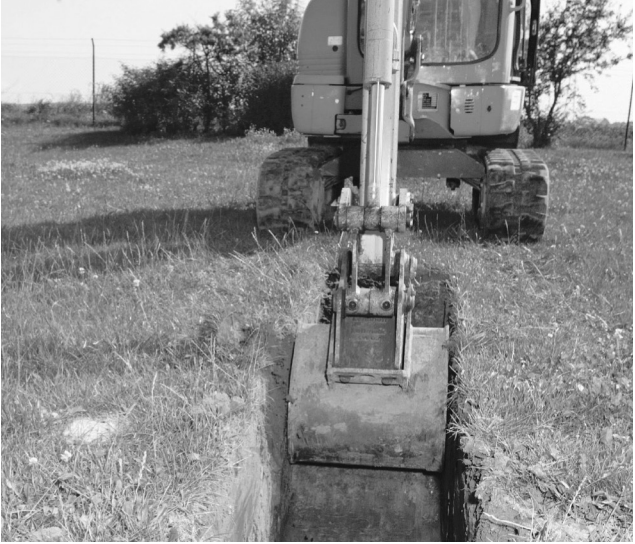
Fig. 5.1: Preparing the trench
