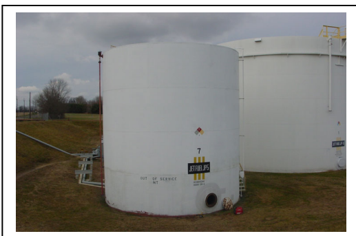
This 30'Ø tank can be inspected using SP001.
