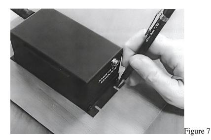
With the brackets now installed, place the intercom into the hole backwards (facing into the panel), and mark the location of the mounting screw holes using the bracket slots as a template as shown in figure 7.
