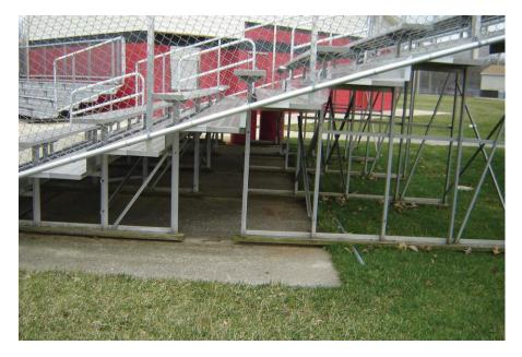
Mudsill, unanchored 10 row x 27' stand blown half off slab,other identical stand blown over and destroyed itself and backstop fence
