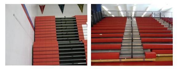
8 ft. wide aisle with single line of centered handrails
