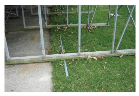
Mudsill stand blown off concrete slab foundation
