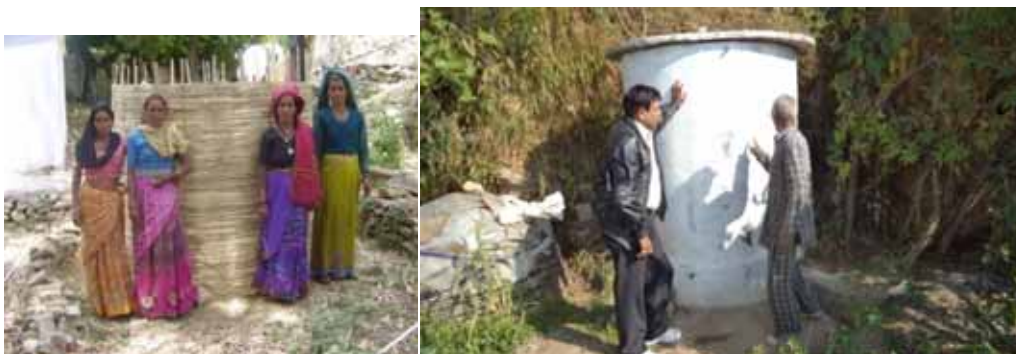
Pictures: Bamboo reinforcement under construction, finished water tank with tap
