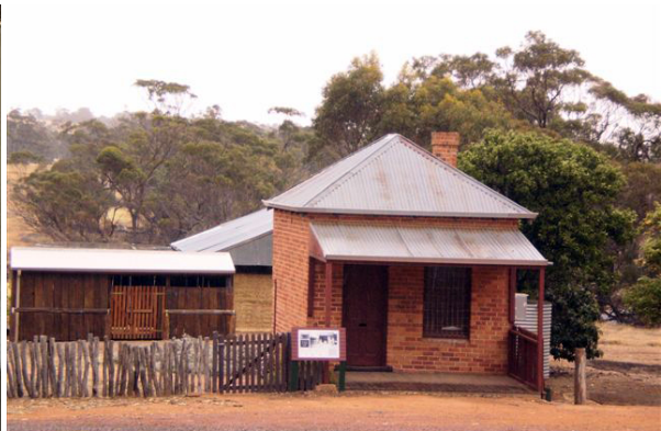
Figure 5: Arthur River Old Post Office
