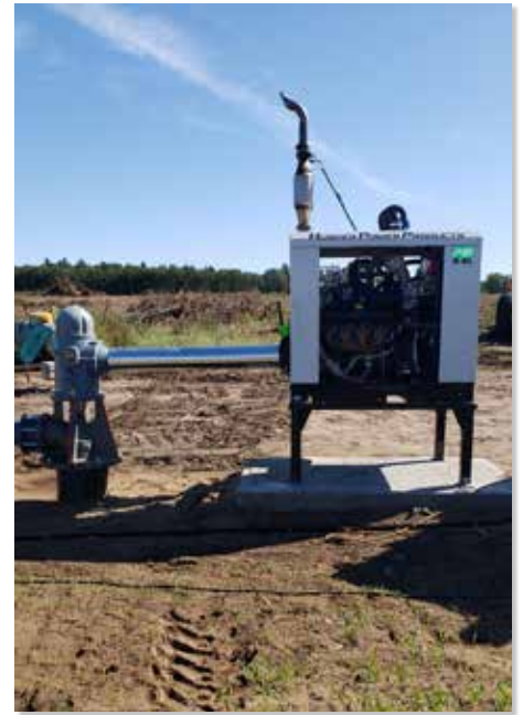
An LP power unit and generator are connected to a turbine pump at Wagner Farms in Adams County, 2019. The design is typically used in locations where three-phase power is not available.
