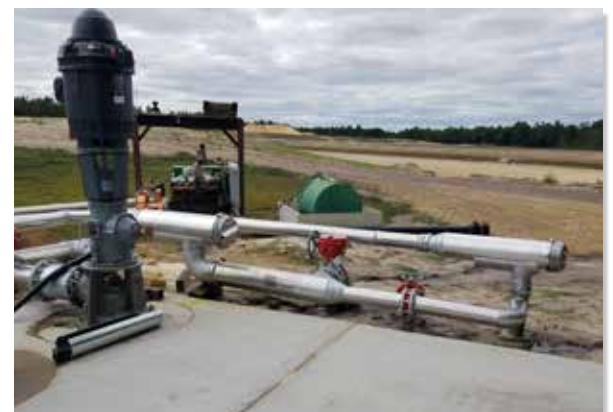
Three variable frequency drives and electric motors power independent turbine pumps at the Wisconsin Cranberry Research Education Foundation, in 2019. The system is fully automated, and if power fails, set up to switch to a diesel backup unit using an automatic combination gear drive.
