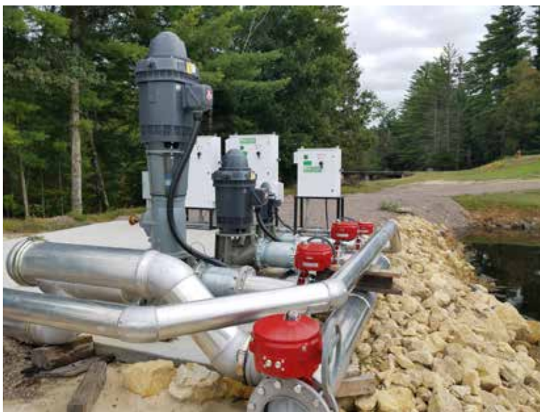
Three variable frequency drives and electric motors power independent turbine pumps at the Wisconsin Cranberry Research Education Foundation, in 2019. The system is fully automated, and if power fails, set up to switch to a diesel backup unit using an automatic combination gear drive.
