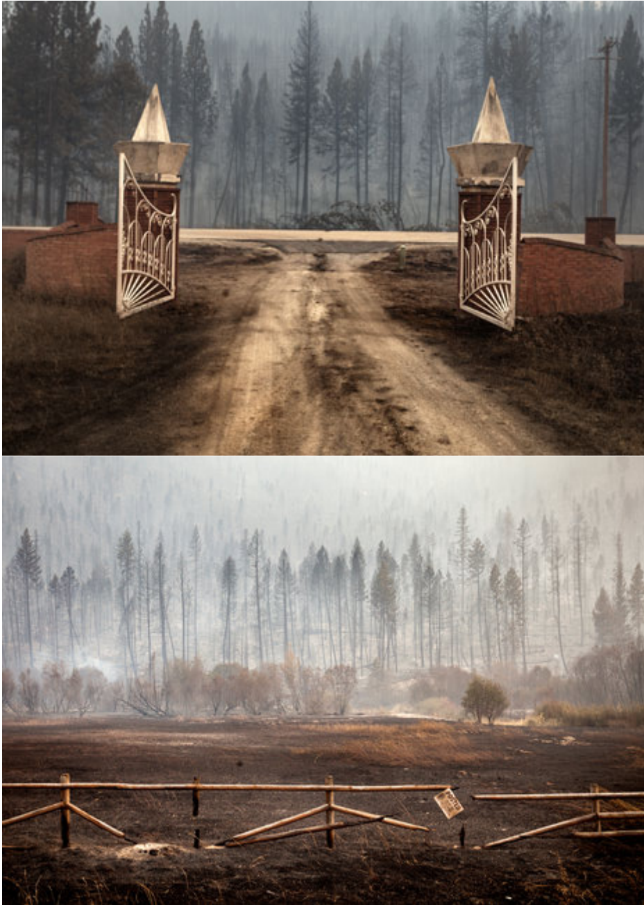
Top: The gate of a house that burned in the Lolo Creek Complex Fire near Missoula. Bottom: Landscape burned along U.S. Highway 12 in Montana.
