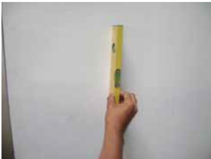
View A. Verify Vertical Leveling
