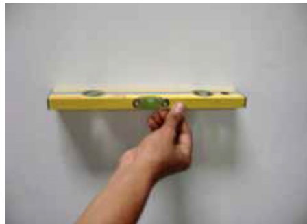
View B. Verify Horizontal Leveling
