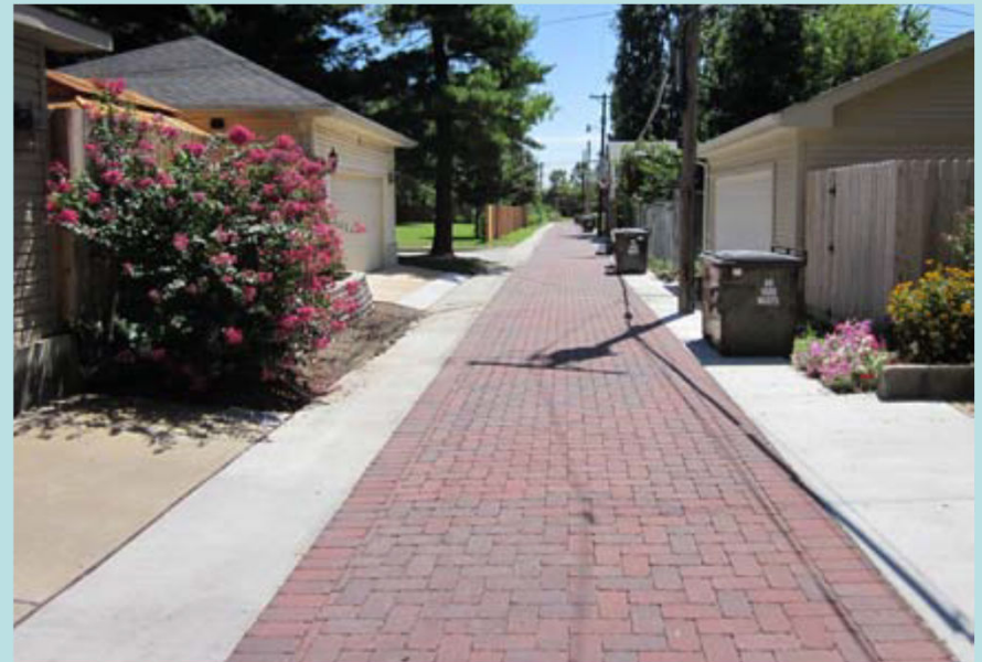
Pervious alley in St. Louis City. Source: Metropolitan St. Louis Sewer District (MSD)
