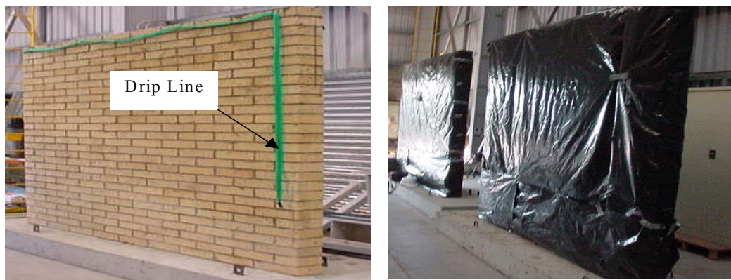
(a) Wall just after construction
