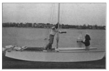
Raise the mast to your shoulder and walk forward with it while extending arms over your head until the mast is held by the side shrouds. NOTE: Make sure to tape the turnbuckle barrel and nuts to prevent them from loosening.
