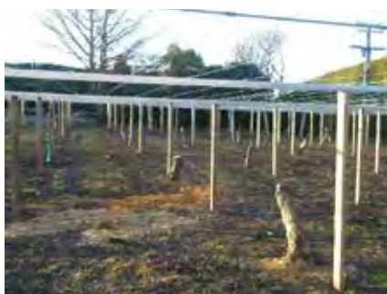
Right: Grafted kiwifruit stumps with pergola structures and wires in place ready for training (Shane Max, Zespri OPC)
